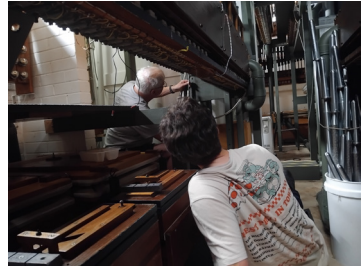
John Weismantel and Oliver Dunk installing the magnet boards
